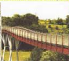
Stressed ribbon bridge
