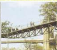
Underspanned suspension bridge
